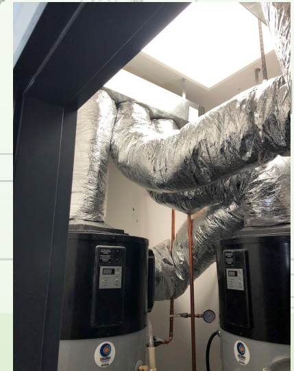
NEGLY AVENUE APARTMENTS - DISTRIBUTED HP HOT WATER HEATERS
