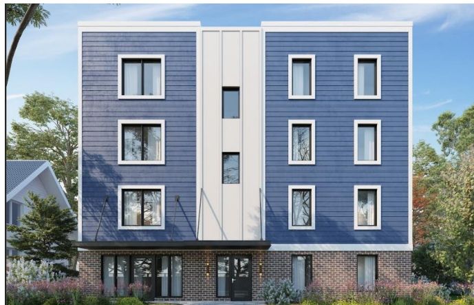
Solstice Northeast (Under Construction)
