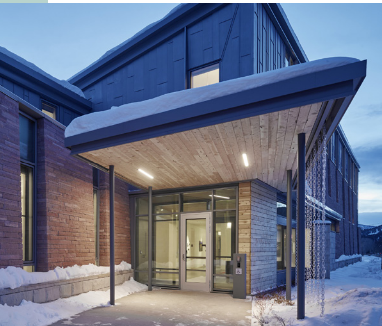
Exterior materials are beautiful, sustainable, and durable. Sandstone walls reflect the surrounding Rocky Mountains, their battered ledges catching snowdrifts. Juniper accents the exterior, lending extreme durability and longevity to the building.
