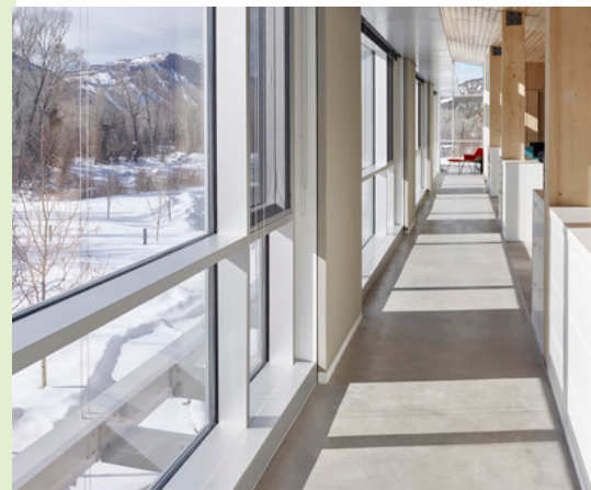
25 The high window-to-wall ratio in the south wall weaves together the view and the energy strategy.
