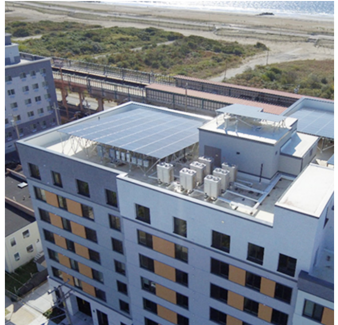
Large buildings are a great fit for PHIUS. Large buildings are easier to make energy efficient, so the cost premium for PHIUS diminishes, too. This apartment building cost about 2 percent more to build than a comparable code building on Long Island, NY.
