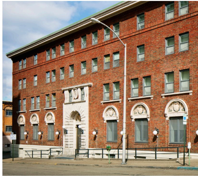
A historic landmark brought into the 21st century. This iconic YMCA building in McKeesport, PA, was retrofitted into SRO housing for homeless people.
