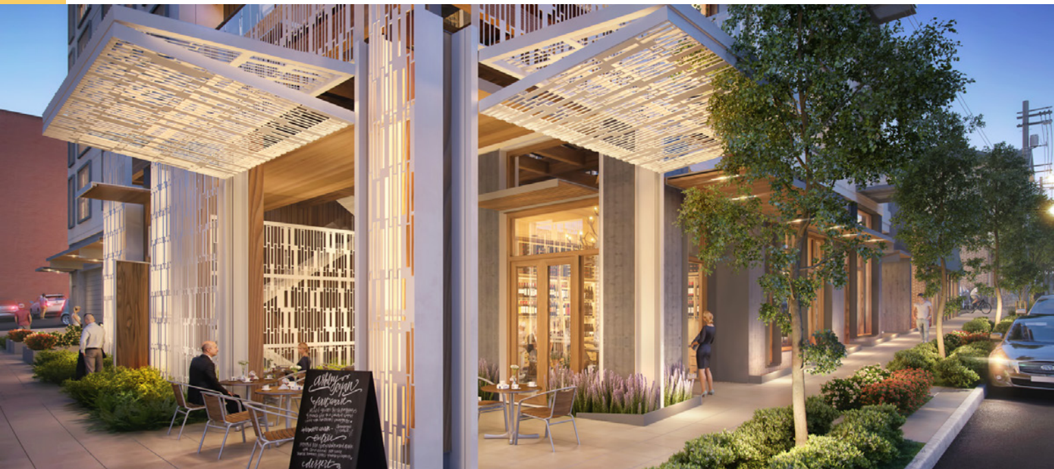
A mixed-use experiment that cost less than 5 percent extra. Seattle's 13th and Pike is a six-story apartment building with 48 units, retail, and a parking garage. The total hard cost was $4.2 million; the PHIUS premium was about $200,000, or 4.75 percent.
