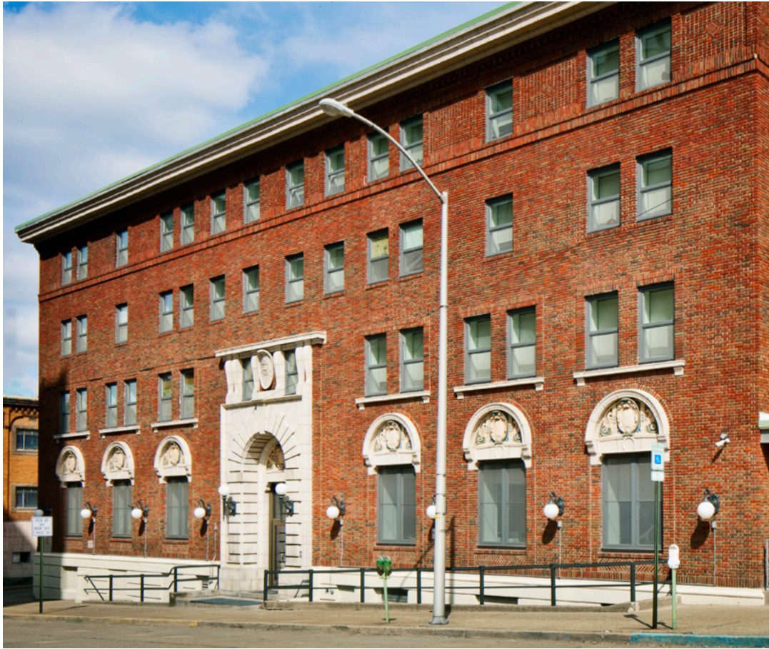
A historic landmark brought into the 21st century. This iconic YMCA building in McKeesport, PA, was retrofitted into single room occupancy housing for homeless people.
