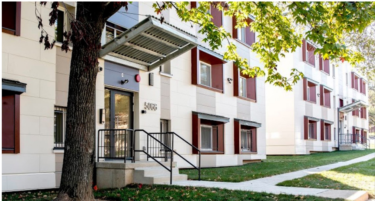
The first multifamily retrofit to earn PHIUS+ certification. The Harry and Jeanette Weinberg Commons, developed by Housing Up and completed in 2015, uses 75 percent less energy than a comparable code retrofit in the Washington, DC, area.
