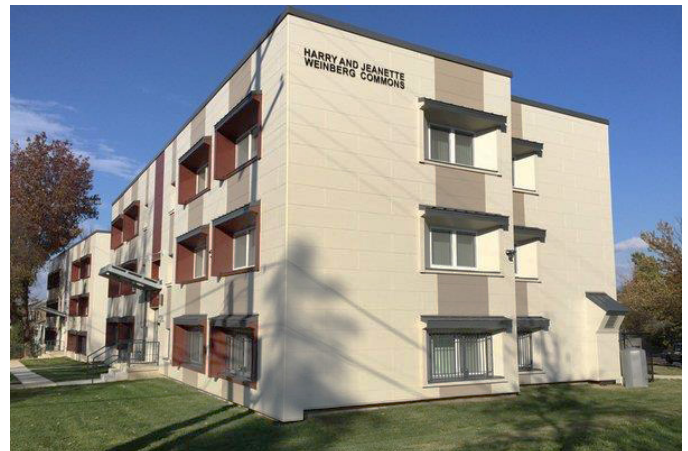
Affordable housing discount. Three foreclosed and vacant properties in Southeast DC were retrofitted into a 36-unit mixed income permanent supportive housing (PSH) community. Developed by Housing Up, it’s the first multifamily passive-building project of its kind in Washington DC.
