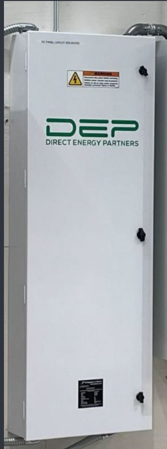
DC POWER DISTRIBUTION PANEL
