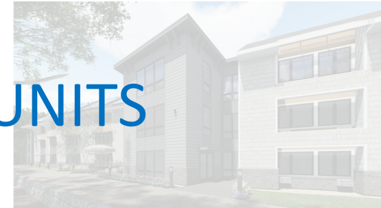
555 MERRIMACK: CONSTRUCTION STARTING 2022
