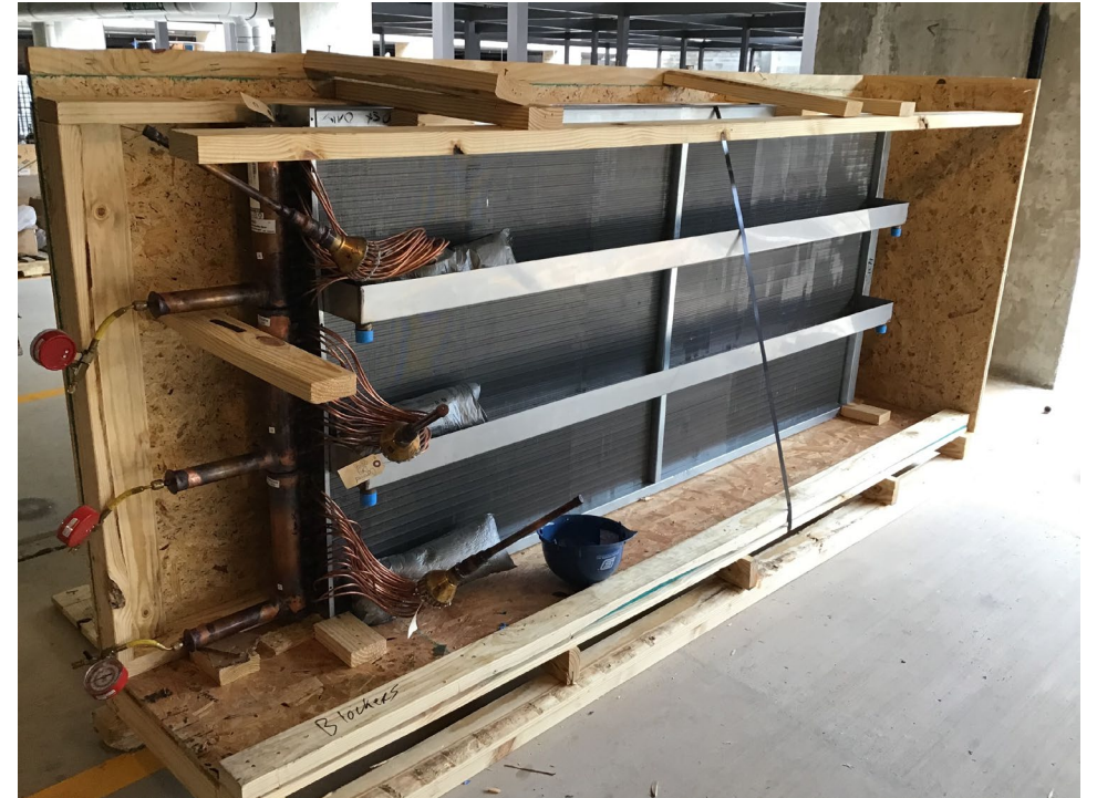
Cooling and Reheat Coils
