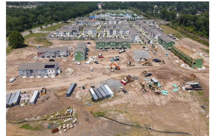
PHASE 3 - IN CONSTRUCTION
