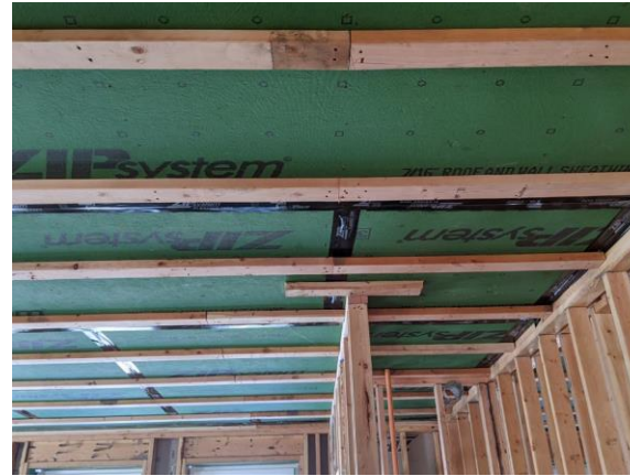
PHASE 1 & 2 CONSTRUCTION PHOTO
