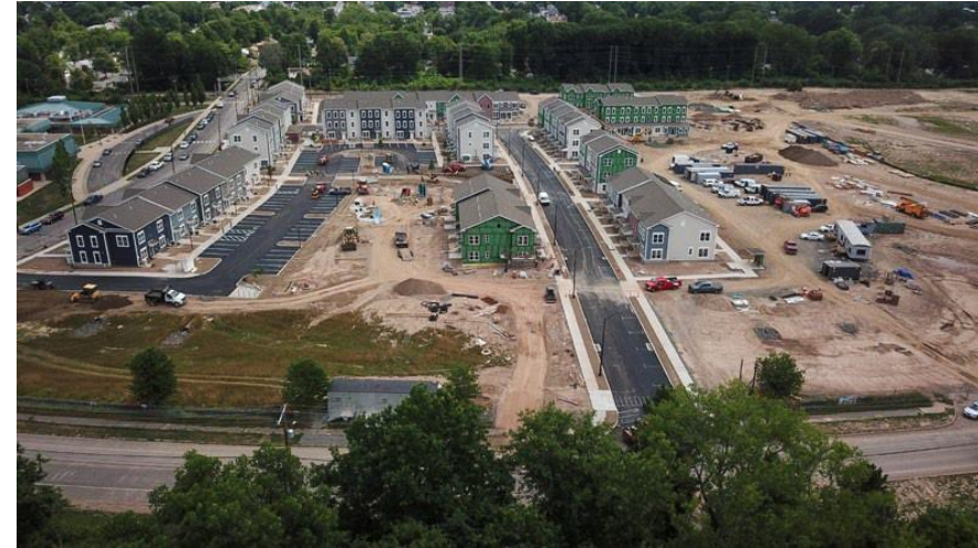
PHASE 1 & 2 - IN CONSTRUCTION
