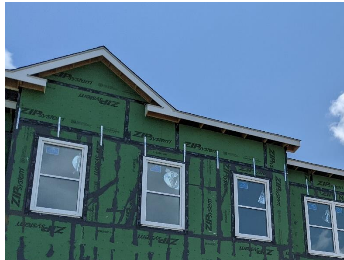
PHASE 3 CONSTRUCTION PHOTO
