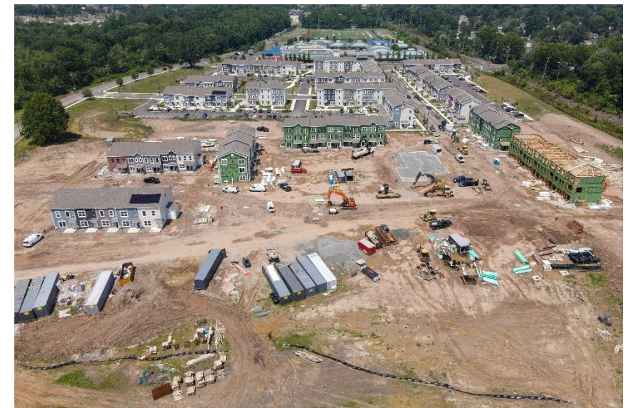
PHASE 3 - IN CONSTRUCTION
