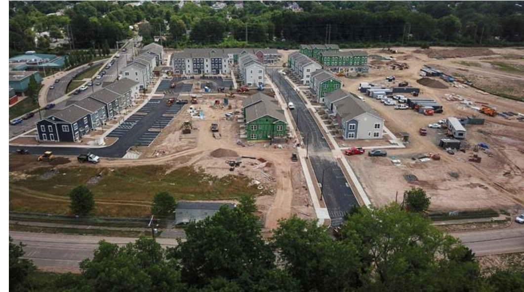
PHASE 1 & 2 - IN CONSTRUCTION
