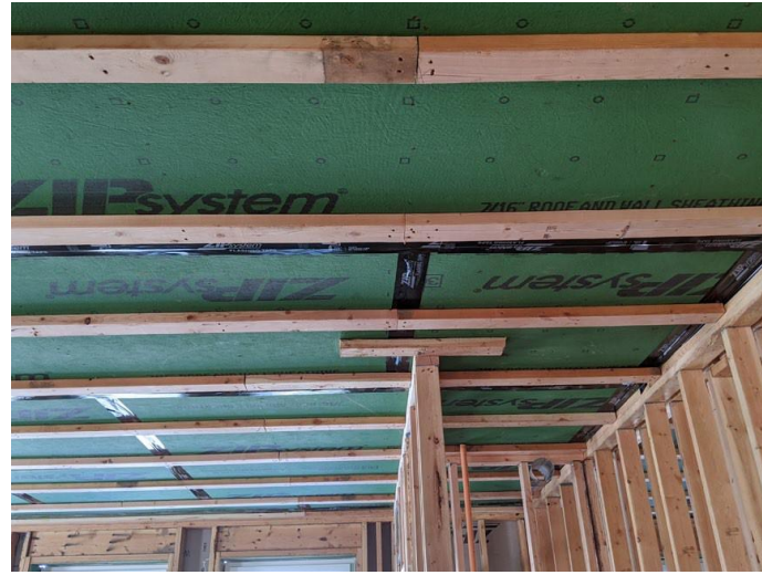
PHASE 1 & 2 CONSTRUCTION PHOTO
