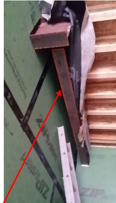
W16x26 Penetrating Thermal Envelope!
