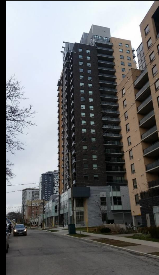
25 story tower Waterloo, Canada
