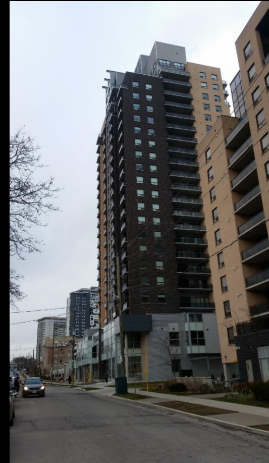
25 story tower Waterloo, Canada
