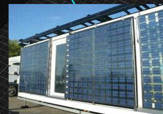
太阳能板预热新风 Integrated Solar thermal system
