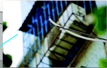
空调凝水回收 Condensing water recycle
