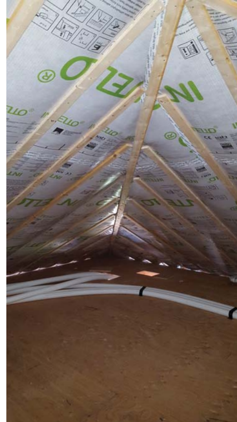
PRO CLIMA 'INTELLO' AIR BARRIER - Air barrier and smart vapor control installed on existing rafters
