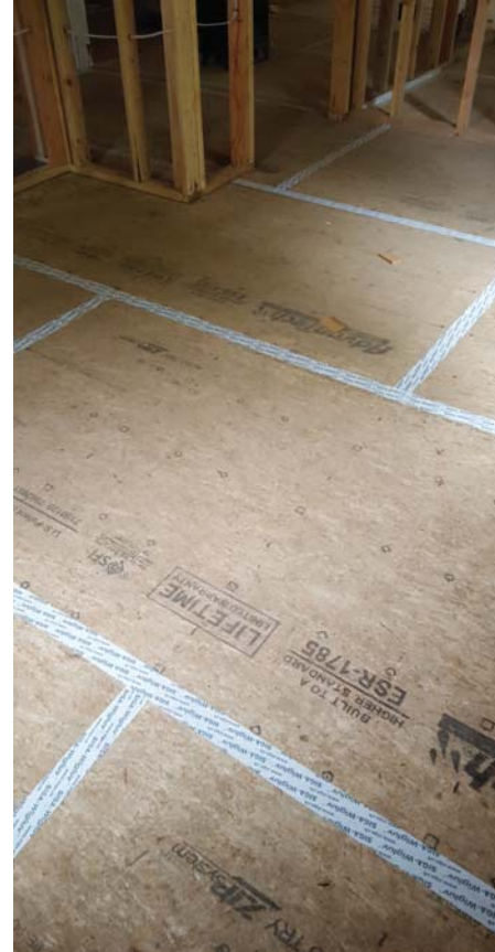
FULLY TAPED OSB SUBFLOOR - a new subfloor is installed and fully taped to create a fail safe in our airtight floor
