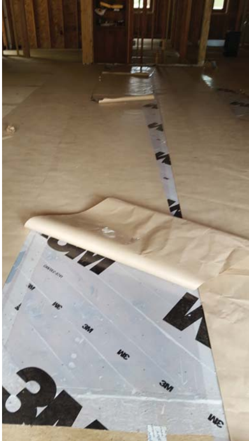
3M '3015' AIR BARRIER - 36" wide rolls overlapping to 'shrink wrap' existing floor and ensure air-tightness on a less-than-ideal substrate
