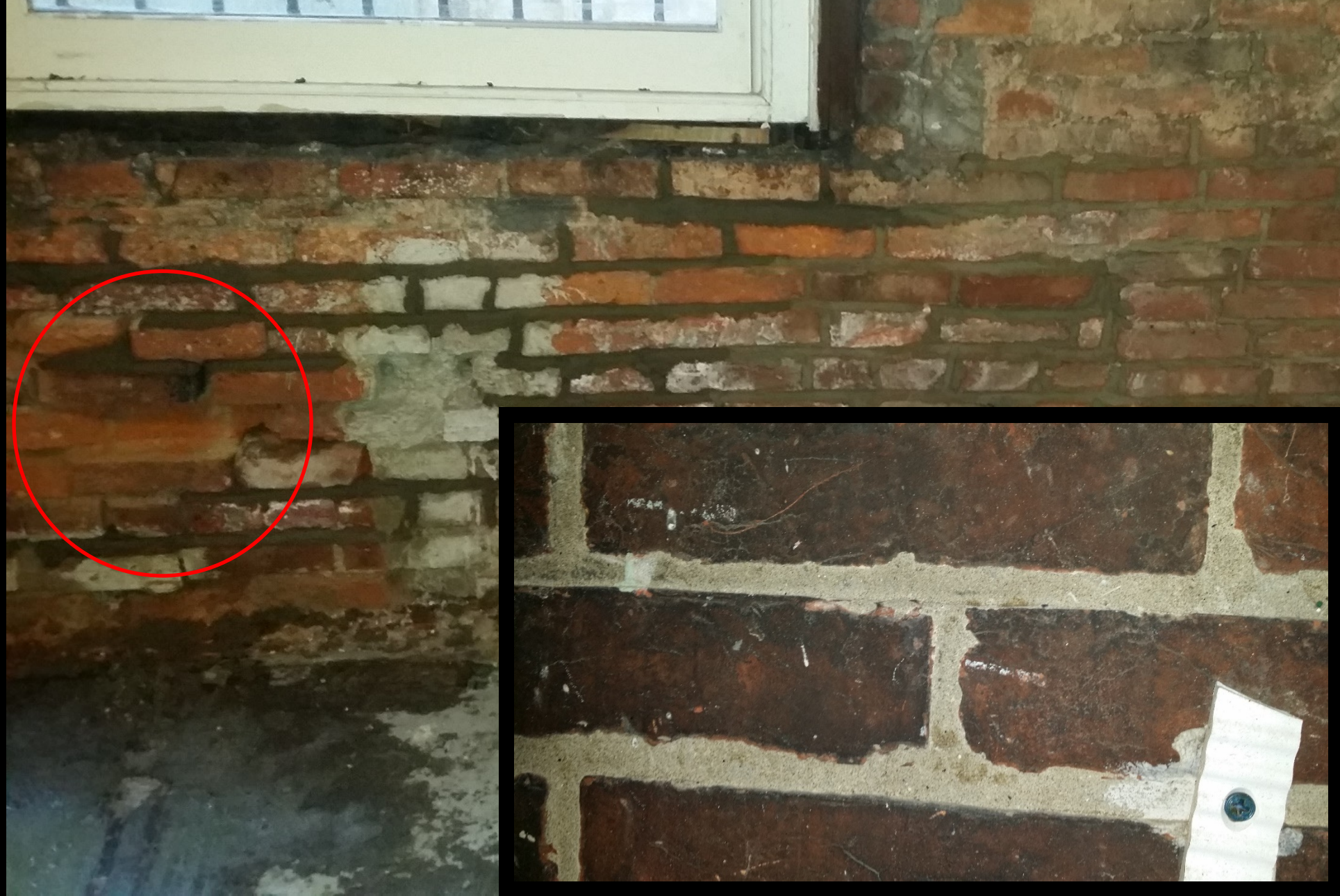
Interior (after pointing)
