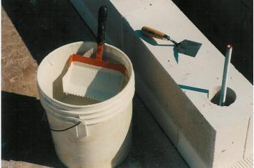
In 1999, the insulation requirement in Maryland for thermal mass walls was R5. AAC alone provided R8. Plaster interior; stucco exterior.
