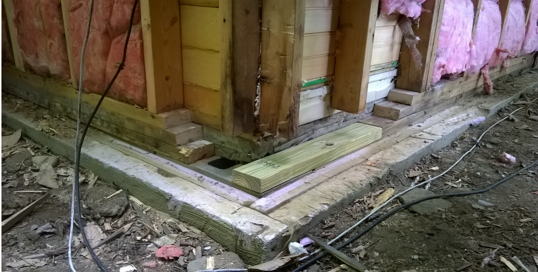
Rear and West wall sill repair
