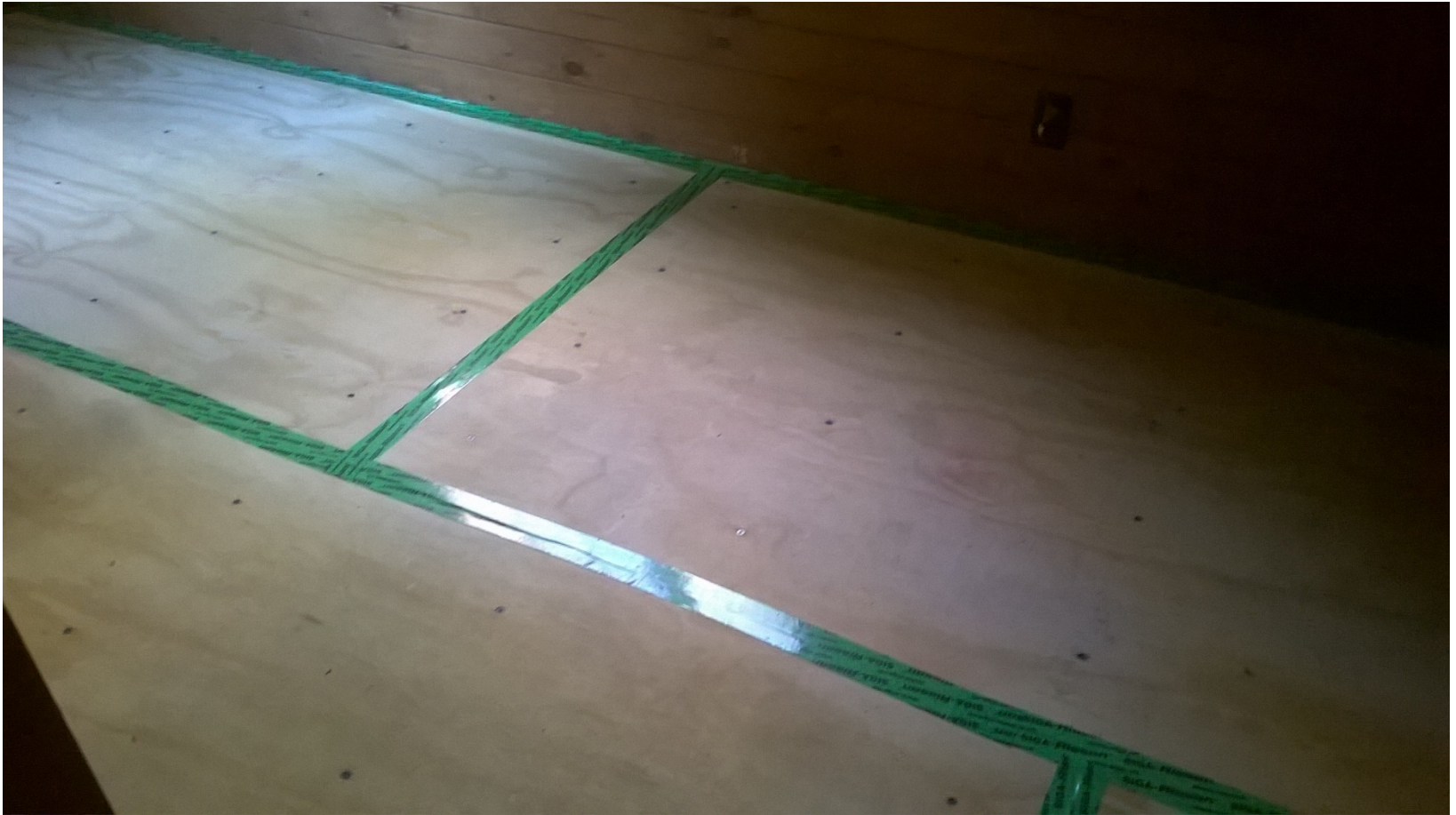
Interior floor plywood over ISO board
