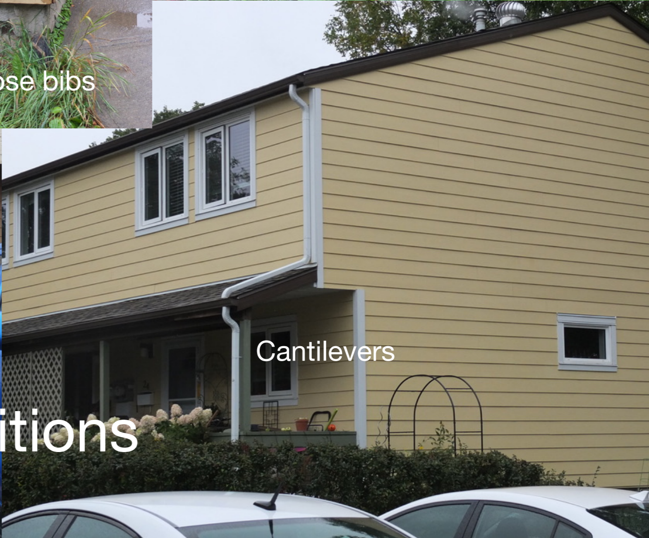
Openings tight to inside corners
