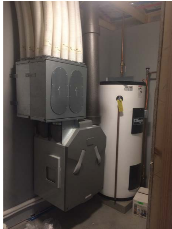
Electric water heater (Vaughn 3" polyurethane foam)
