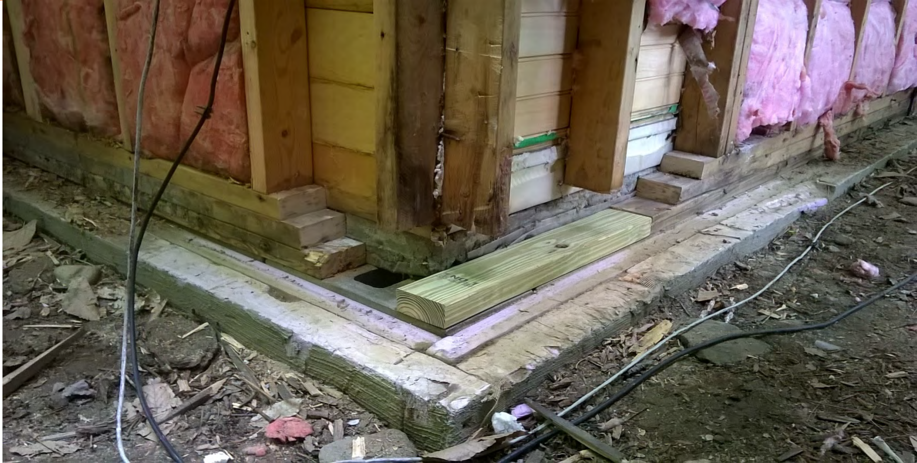
Rear and West wall sill repair
