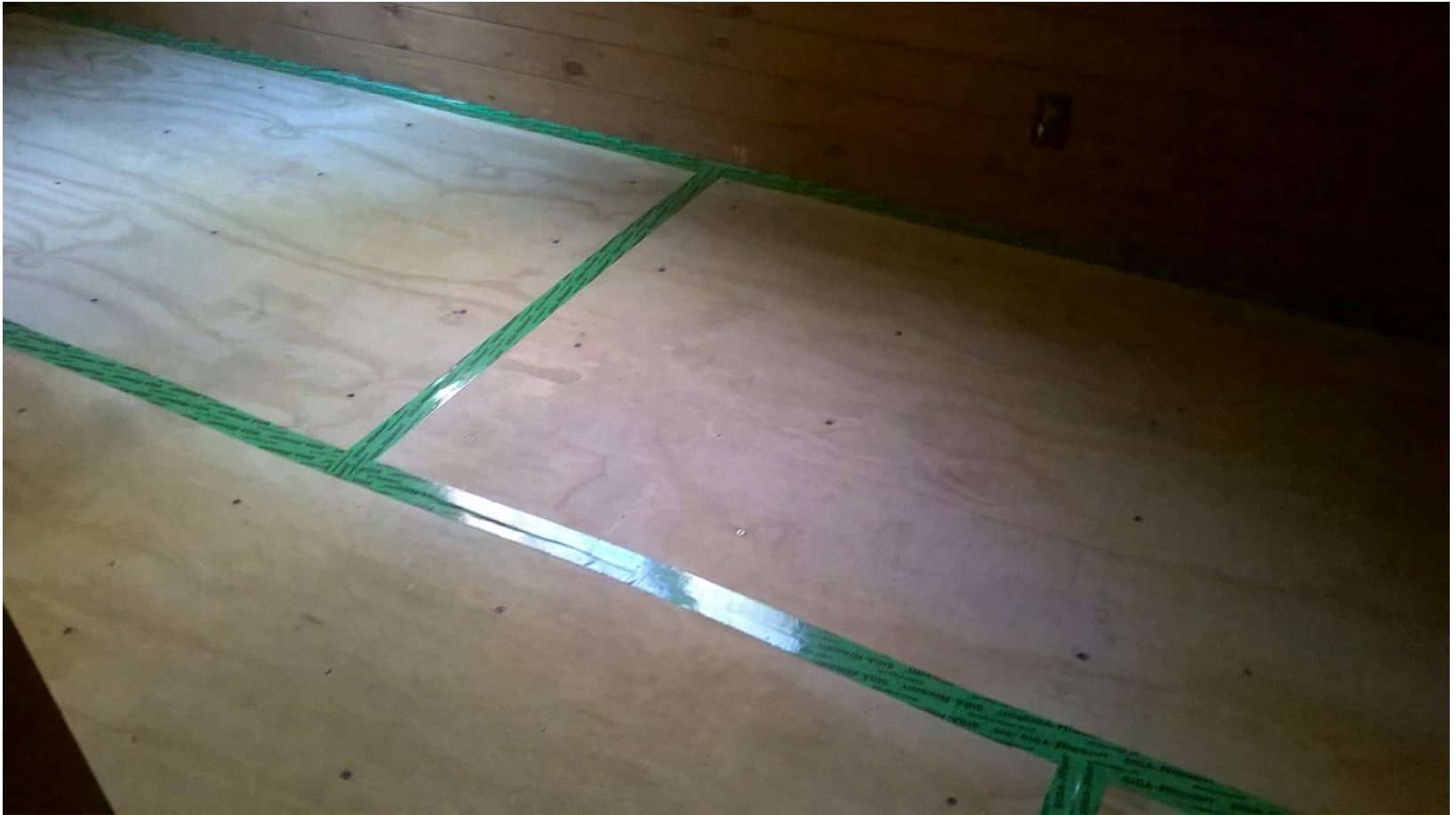
Interior floor plywood over ISO board
