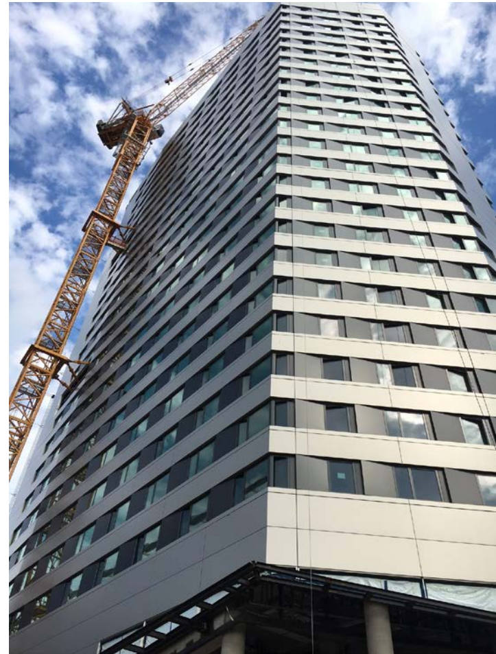
Cornell Tech Building
