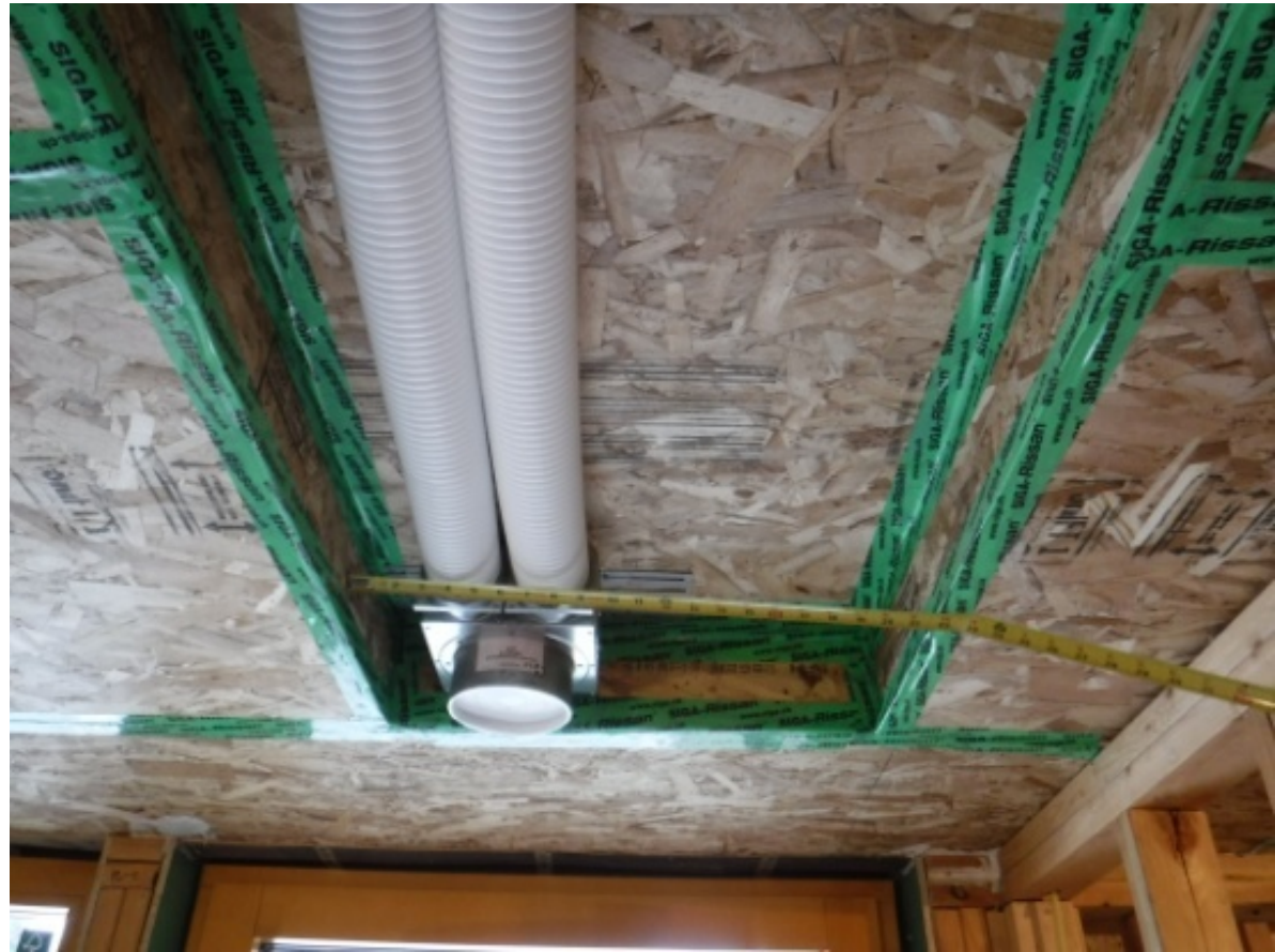
Sealed chase way in truss bay
