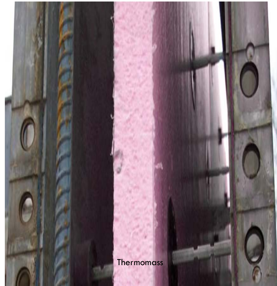
Double Concrete Wall with Sandwich XPS
