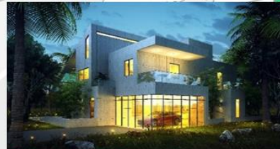
Zhuhai Exhibition Center Gree Nearly Zero-Energy Experience Center
