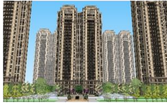
Hebei Residential Building Train City 340,000 m 2
