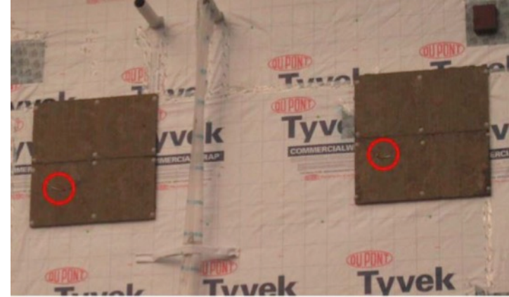
2. RH/T sensors on exterior of mineral wool insulation
