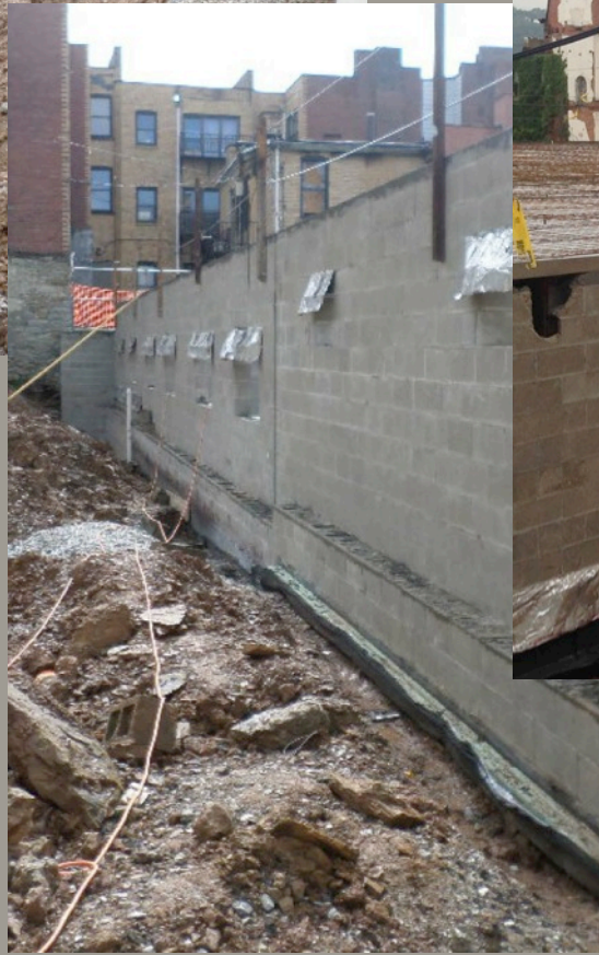
Wall Construction Transition at Grade
