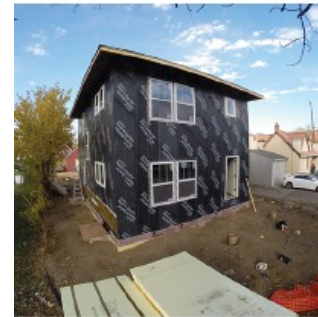
Week 1, house water tight
