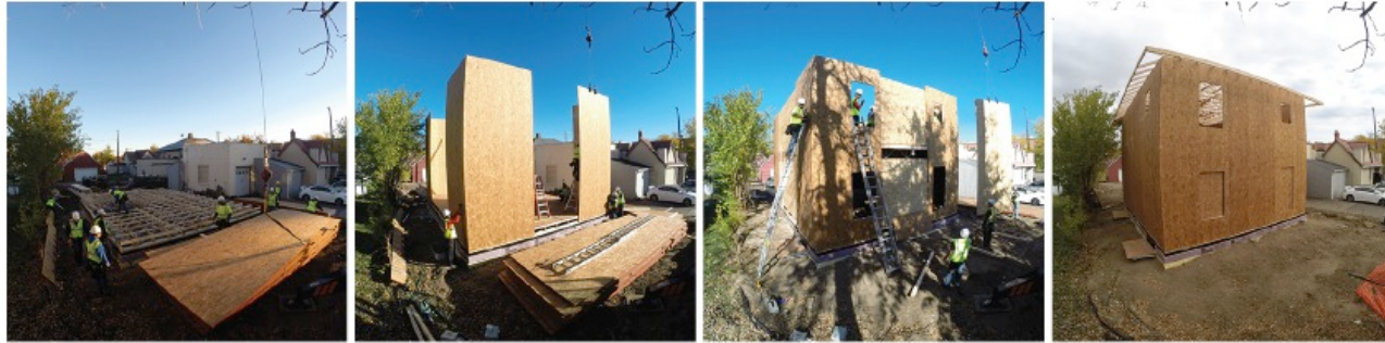
Day 1, structure complete
