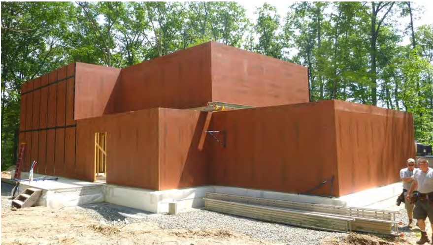
Northwest view of ZIP sheathing over 2x4 frame
