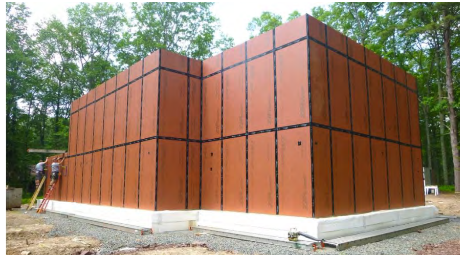
Southeast view of ZIP sheathing over 2x4 frame
