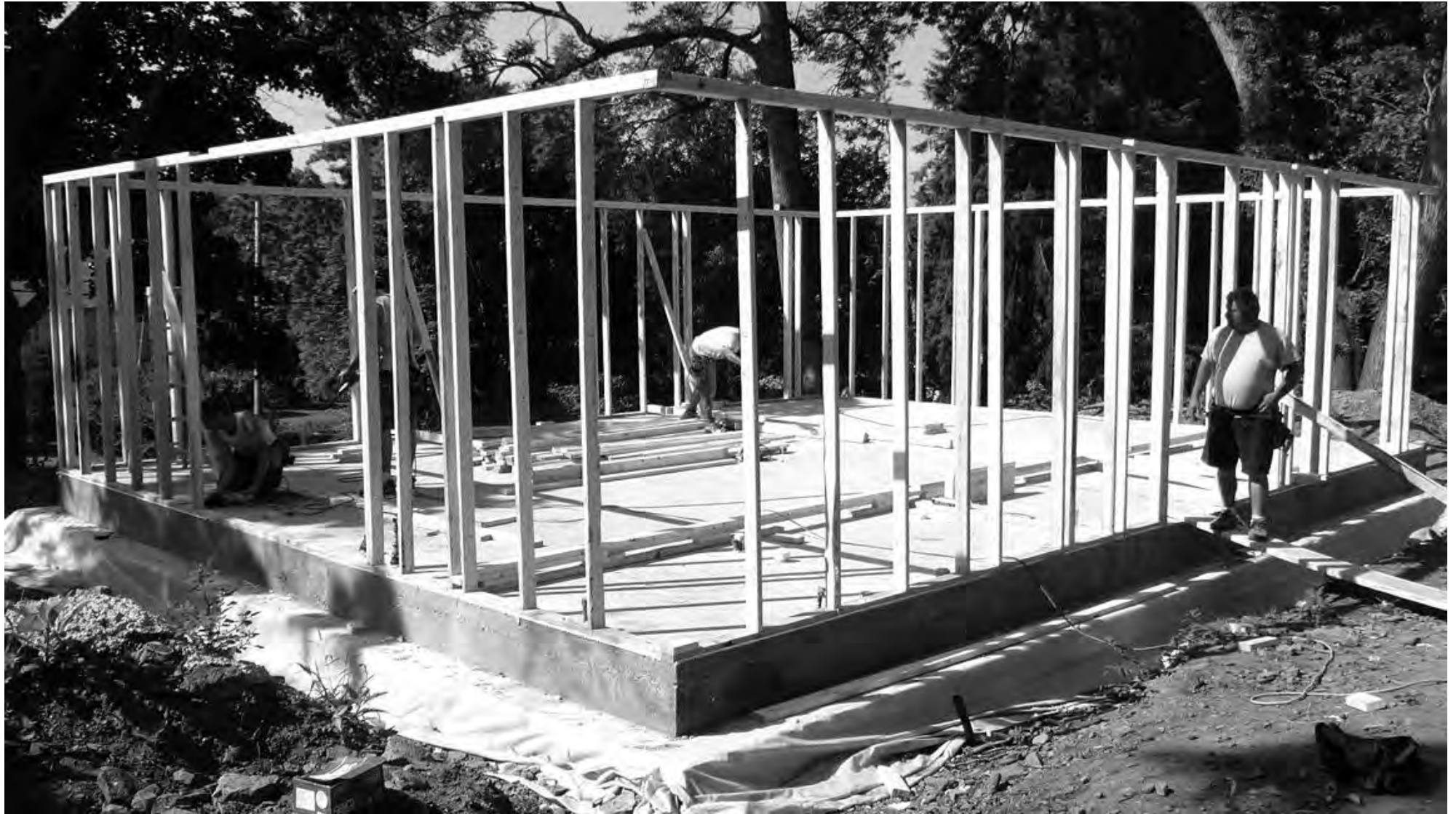
2x4 OVE structural frame
