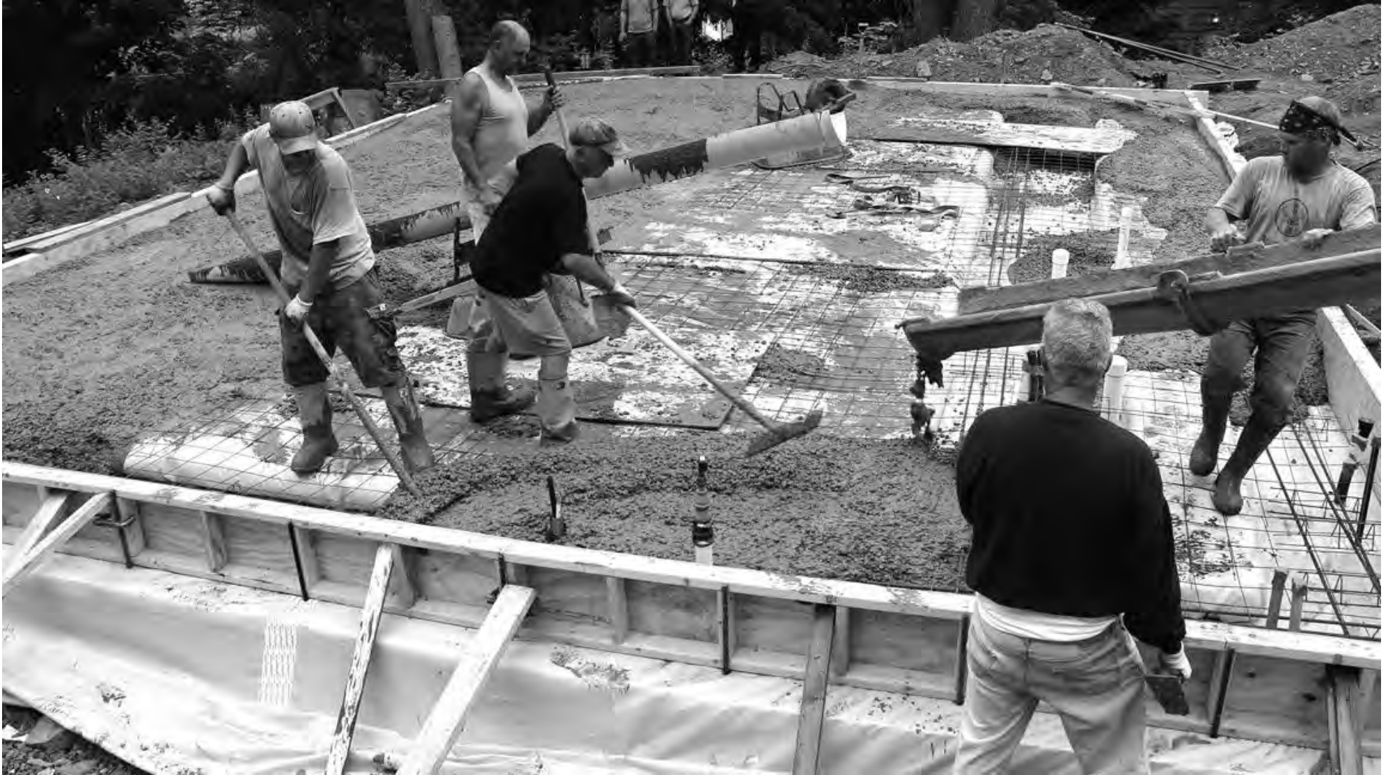
Pouring concrete floor slab over 8" perlite and 12" of EPS Type 9 foam
