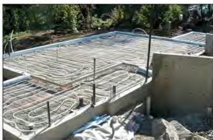
Below: compacted gravel and hydronic heating tubing in place over perlite bag insulation; ready to pour the concrete floor.
