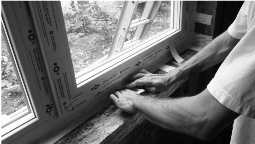
Taping window interior
