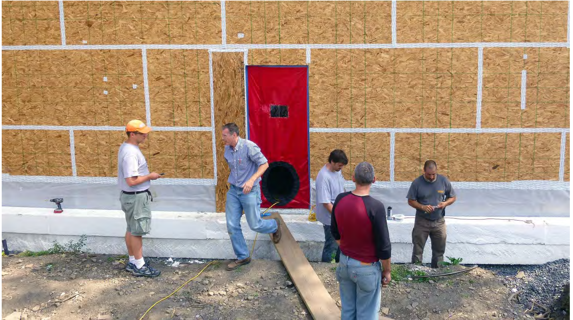
Preparing to positive test exterior after failed negative pressure test
