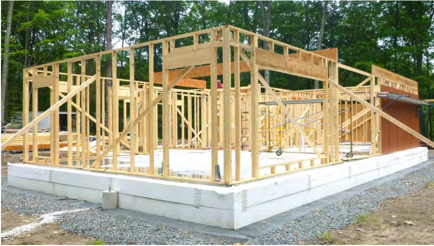
First floor 2x4 framing at 24" O.C.
