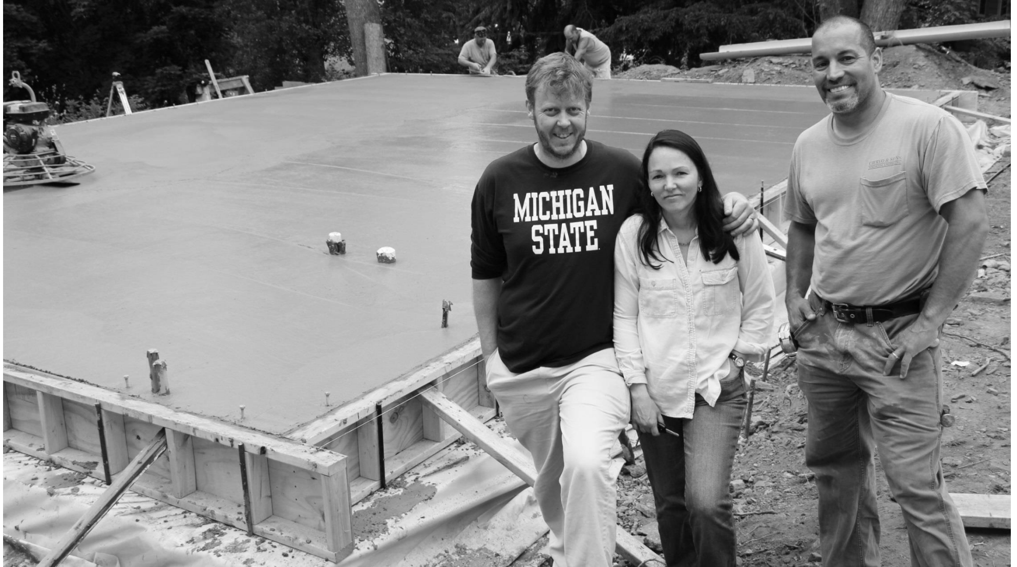
Homeowners Christie and Declan with contractor Rob Ciervo
