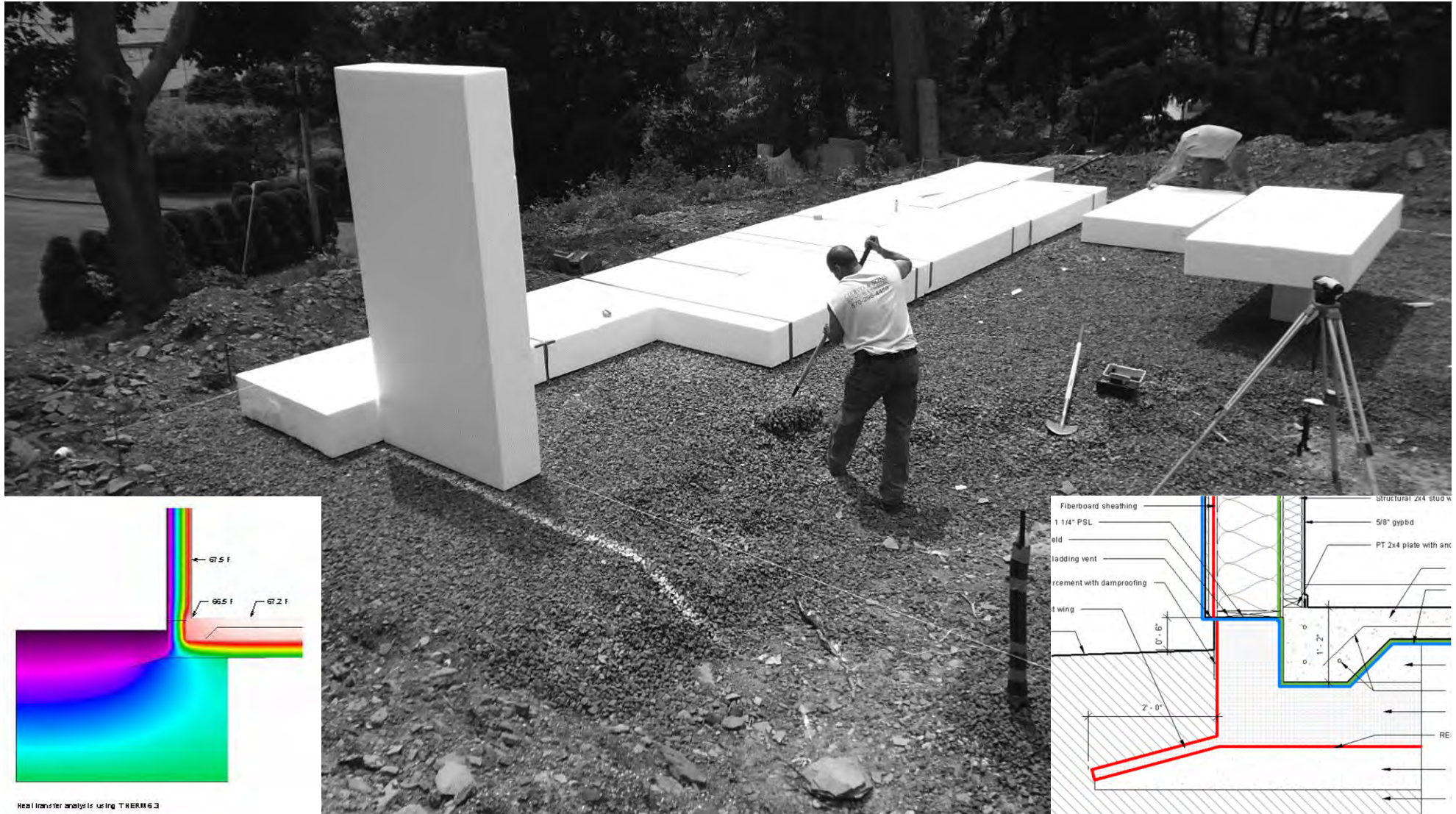
Installing 12" EPS foam over gravel setting bed
