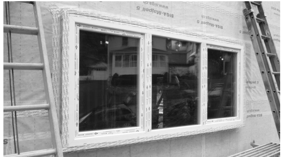
Completed window installation
