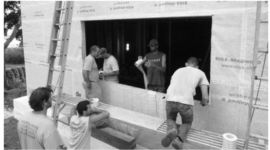
Preparing window exterior
