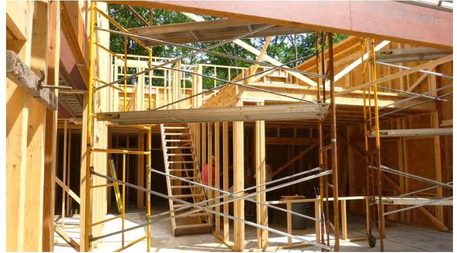
First floor framing at entry
