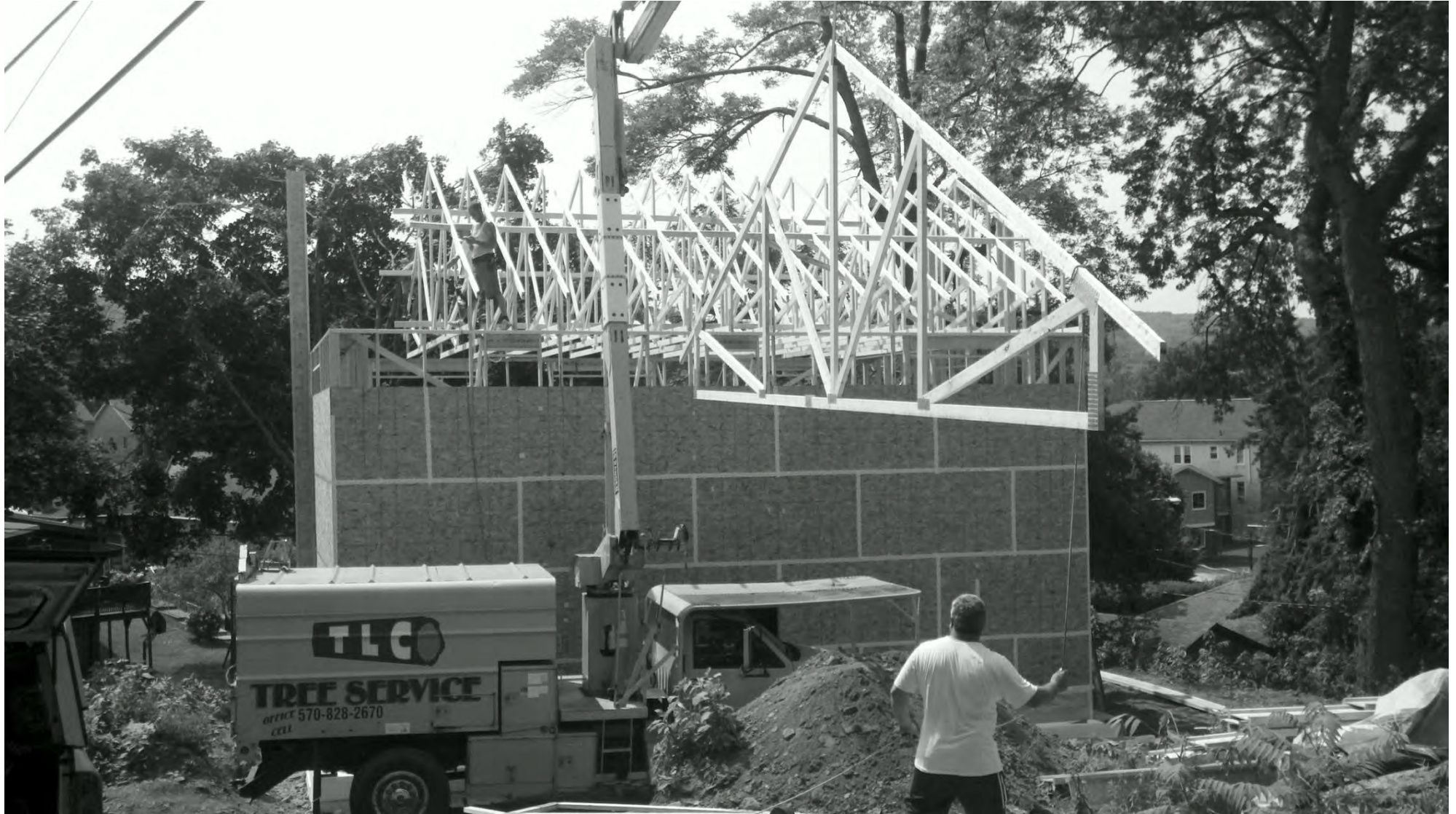
Setting raised heel roof trusses
