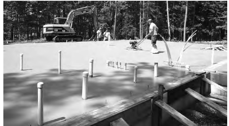
Completed slab with plumbing in place
