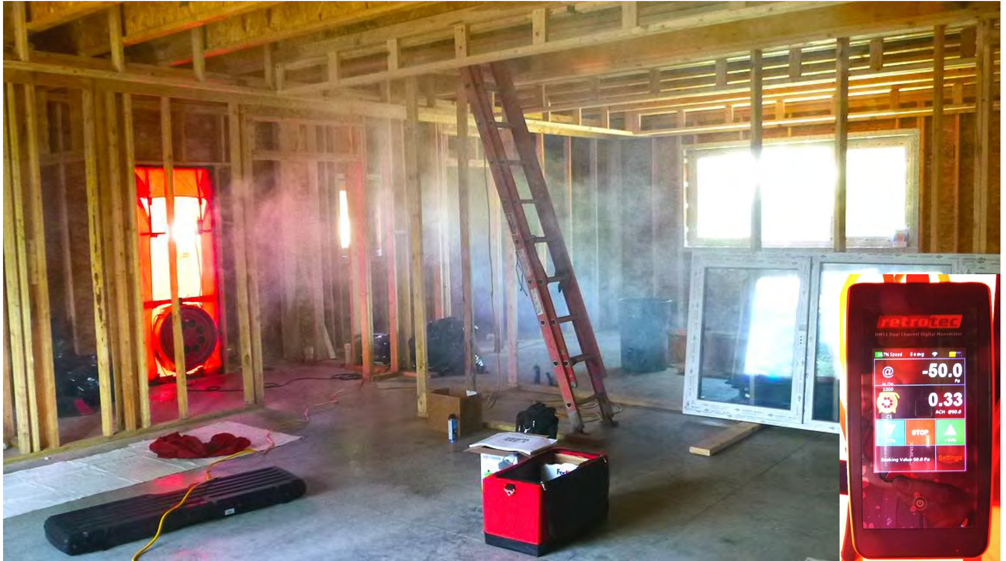
Second blower door test with first window installed
