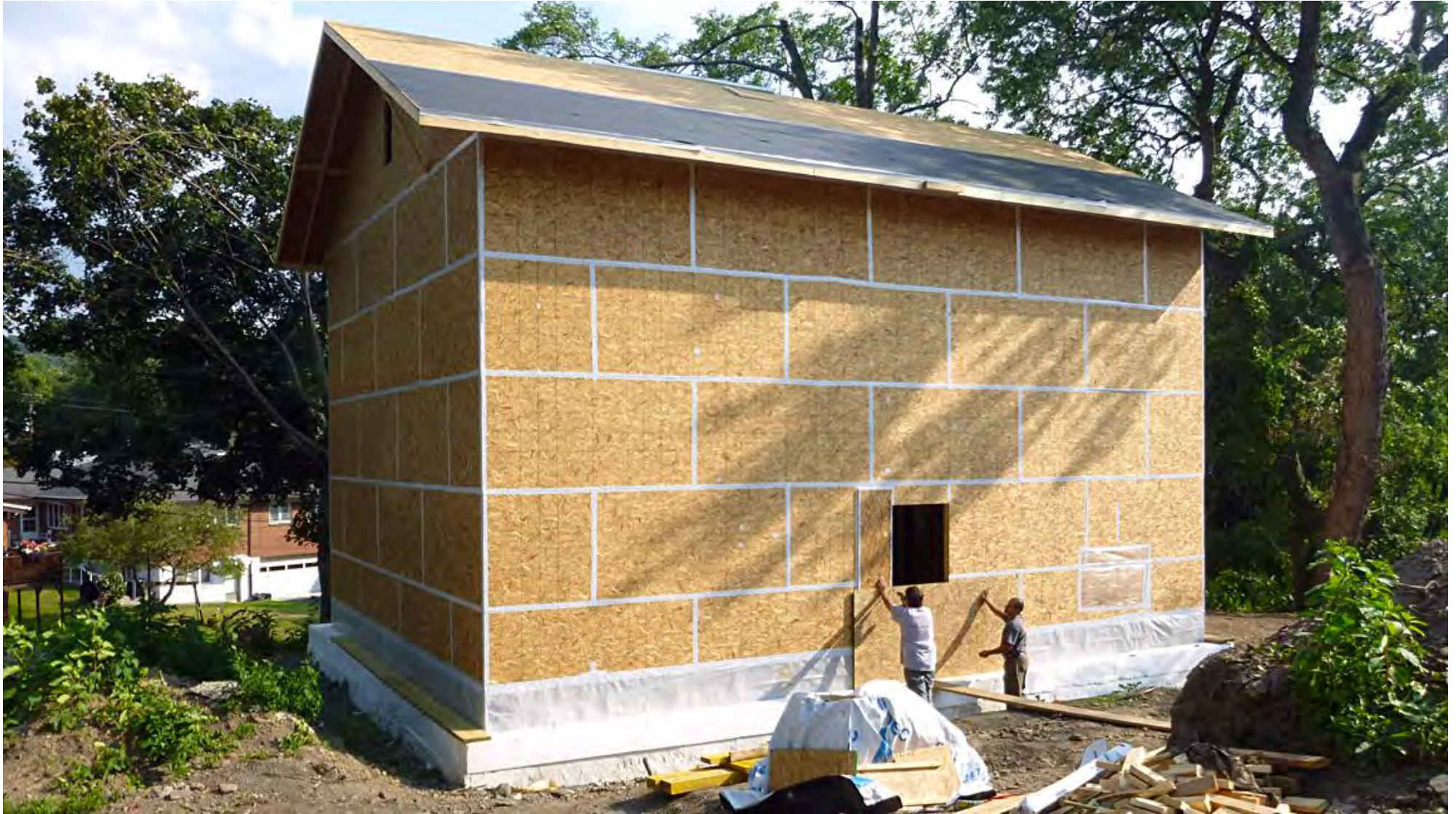
Sheathed and ready for blower door test #1
