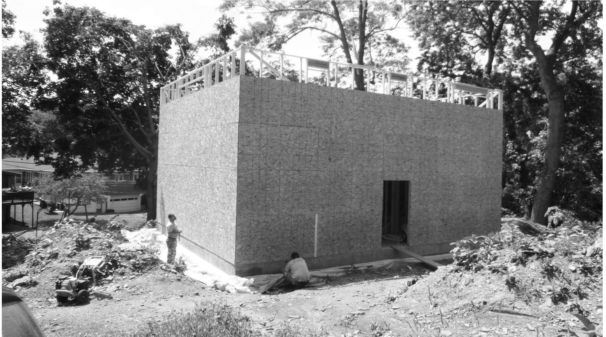
OSB sheathing over 2x4 structural frame with entry door opening
