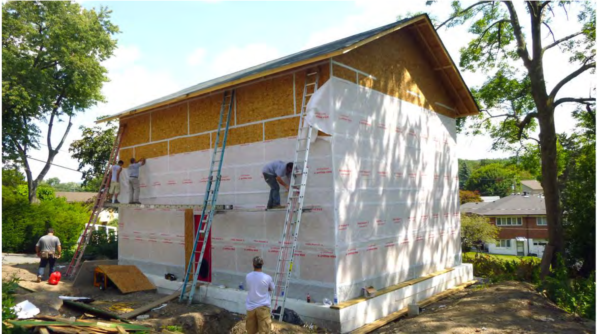
Installing SIGA Majpell 5 on exterior
