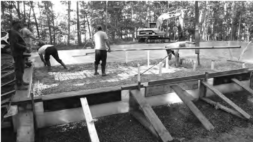
Pouring slab over perlite and EPS foam
