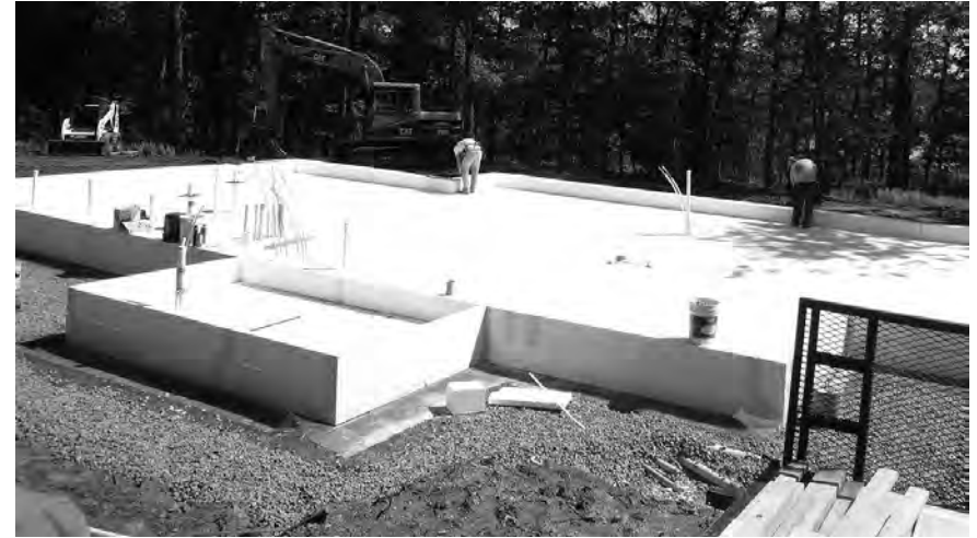
12" of EPS under slab foam
