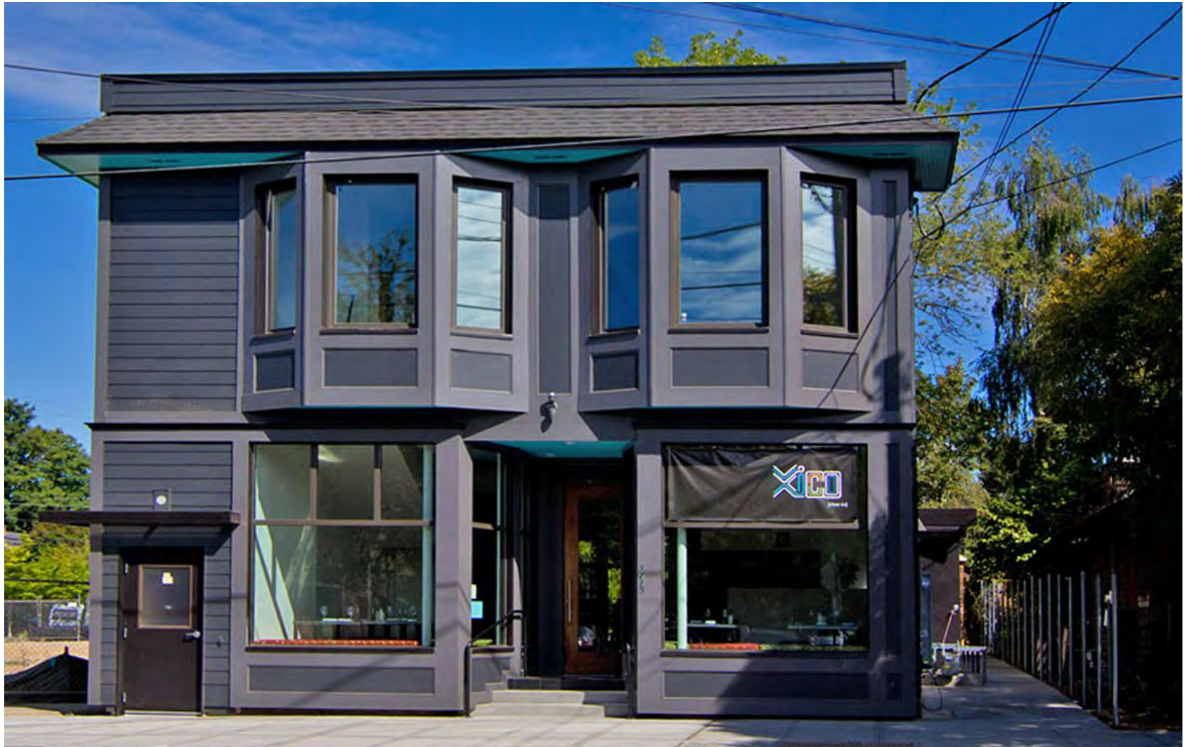
Passive House retrofit of a commercial building
