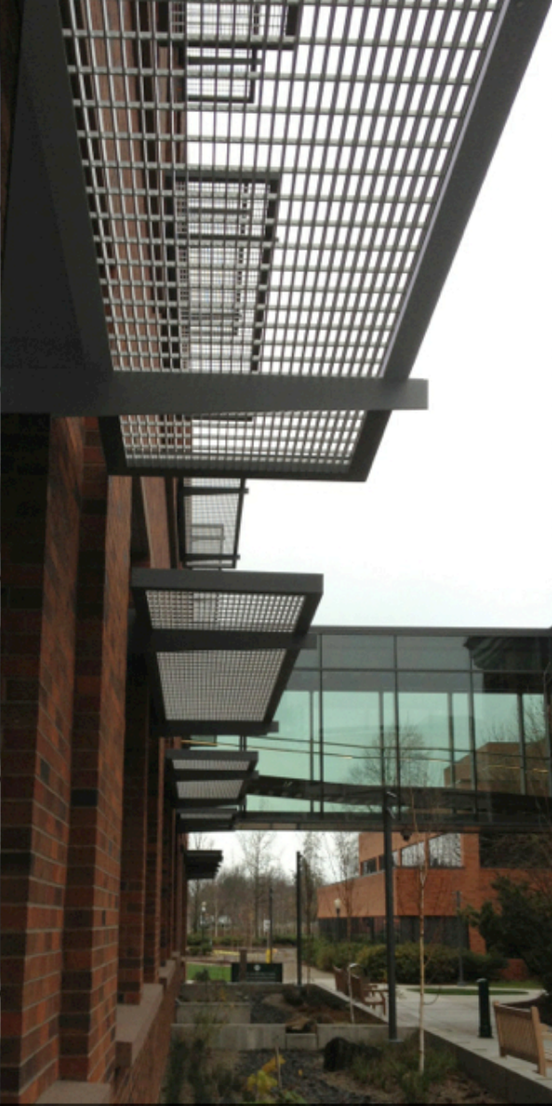
INTEGRATIVE SCIENCE cantilevered steel frame with steel mesh inset
