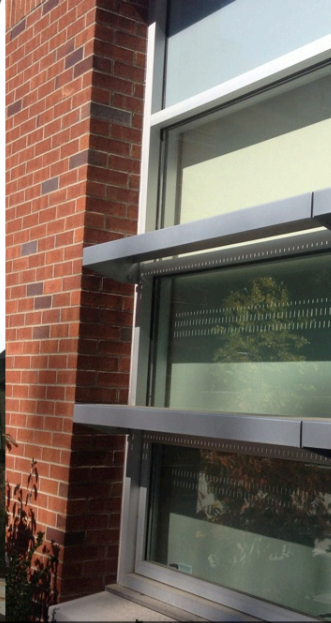
ALLEN HALL mullion-attached, perforated aluminum plates
