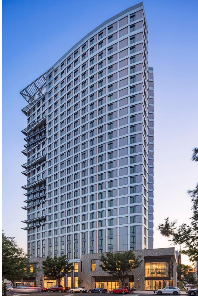
425 Grand Concourse – Dattner Architects (26 stories)
