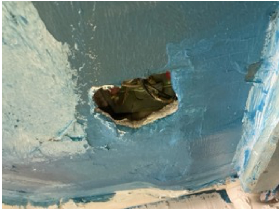
Seal/Cap off or Remove Old Electrical Boxes
