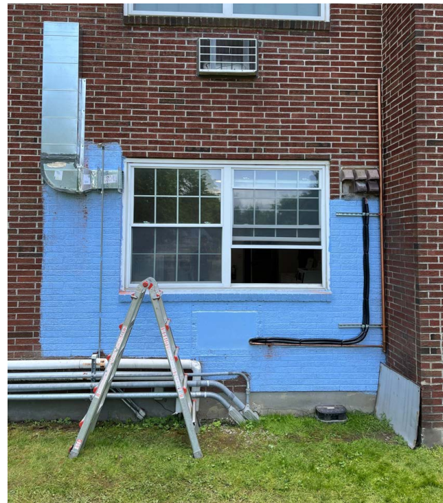
HVAC MOCK-UPS, IN PROGRESS
