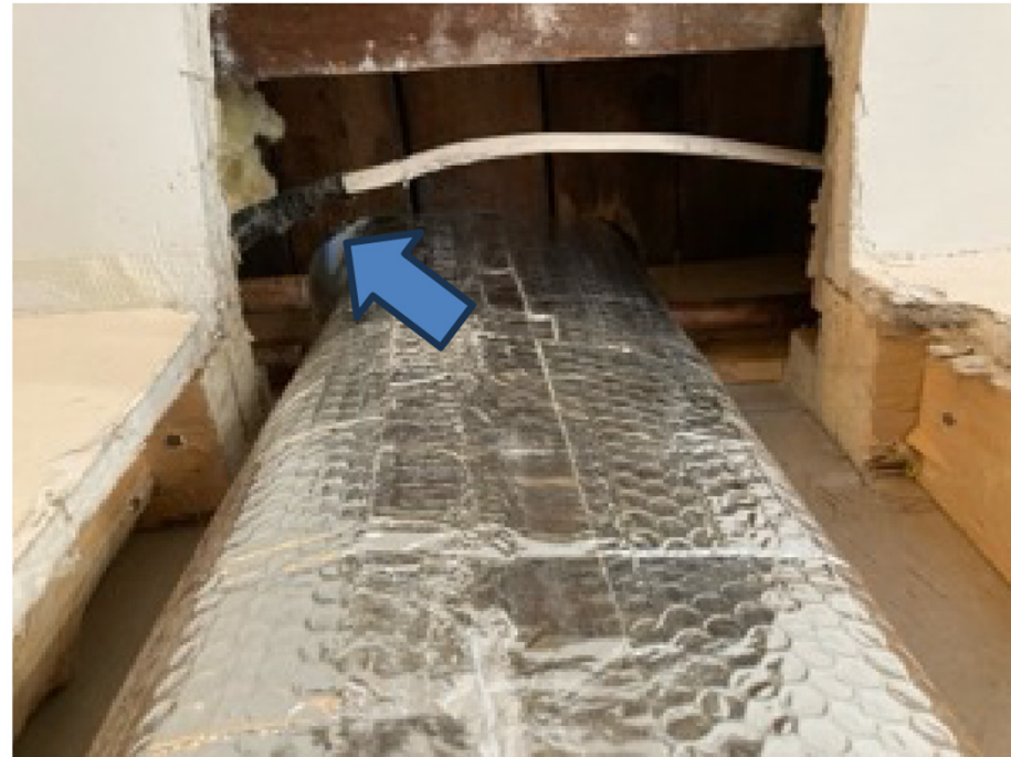
Seal Penetrations In-Between Units
