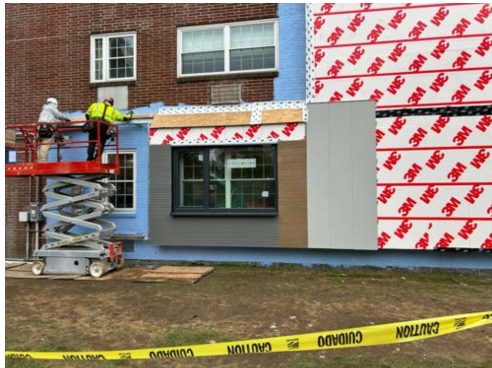
PANELIZED WALL SYSTEM MOCK-UP, IN PROGRESS
