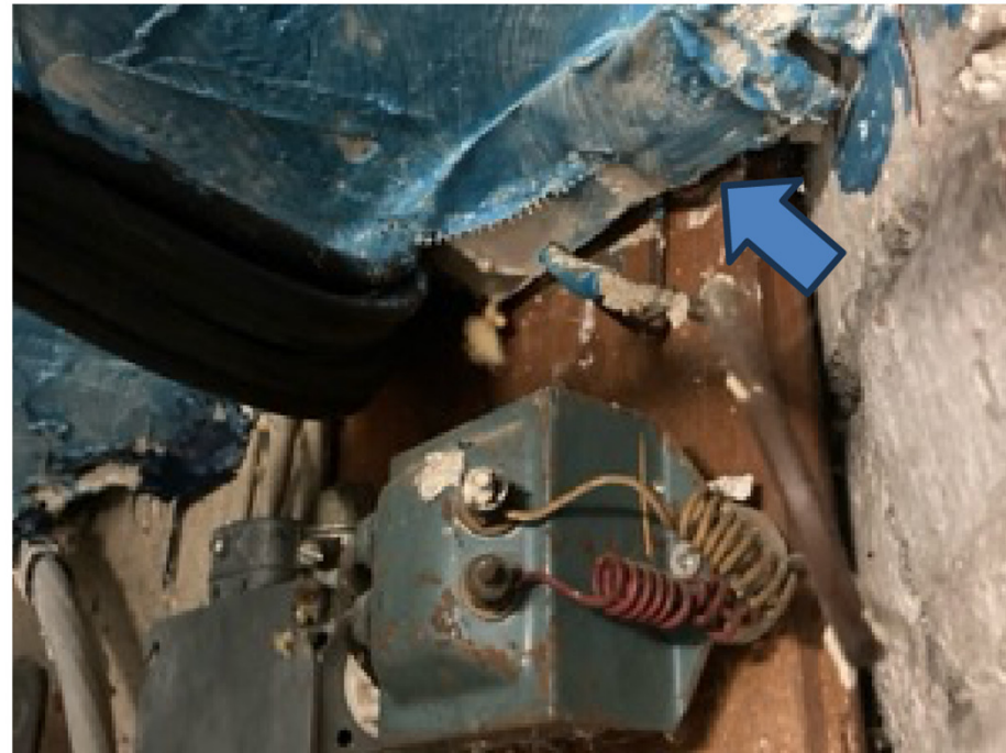
Seal Basement Ceiling Back to the Air Barrier
