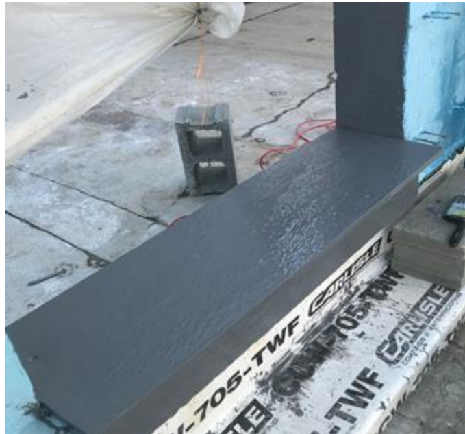
Fluid-applied air barriers at exterior walls (GE Elemax, Henry Air-Bloc All-Weather STPE/31 MR/06 WB, Dryvit NTX and Liquid Flashing)
