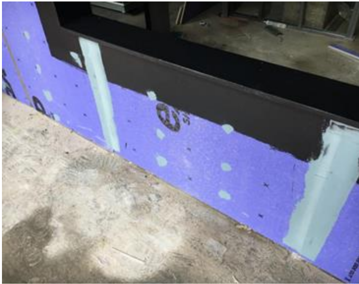
Air-barrier applied to holes and seams before full coat
