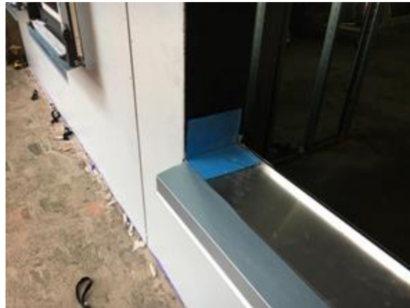
Flexible membrane at sill to jamb transition
