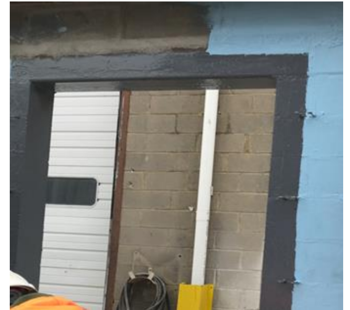
Fluid-applied air barriers at exterior walls (GE Elemax, Henry Air-Bloc All-Weather STPE/31 MR/06 WB, Dryvit NTX and Liquid Flashing)
