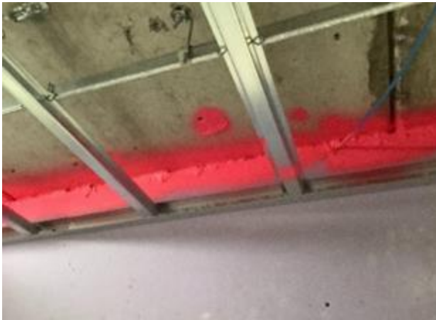
Partition wall firestopping
