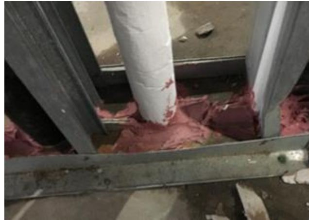
Firestopping at plumbing penetrations
