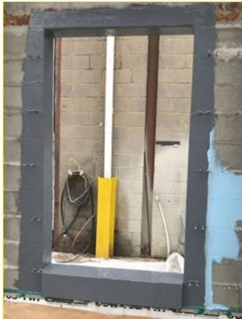
Fluid-applied air barriers at exterior walls (GE Elemax, Henry Air-Bloc All-Weather STPE/31 MR/06 WB, Dryvit NTX and Liquid Flashing)
