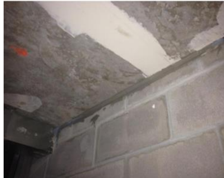
Interior wall and ceiling joint sealing
