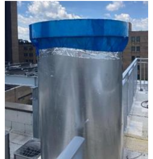
Laundry chute temp. seal
