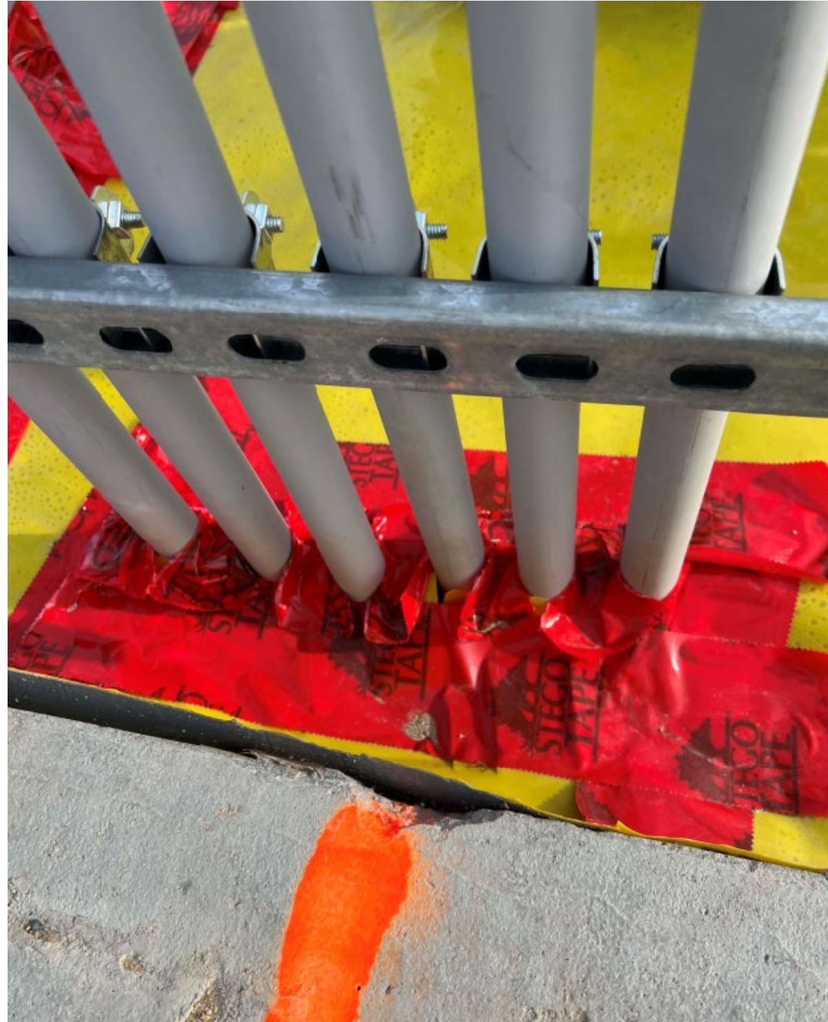
There are different products for sealing the vapor barrier. Conduit and plumbing penetrations require coordination.
