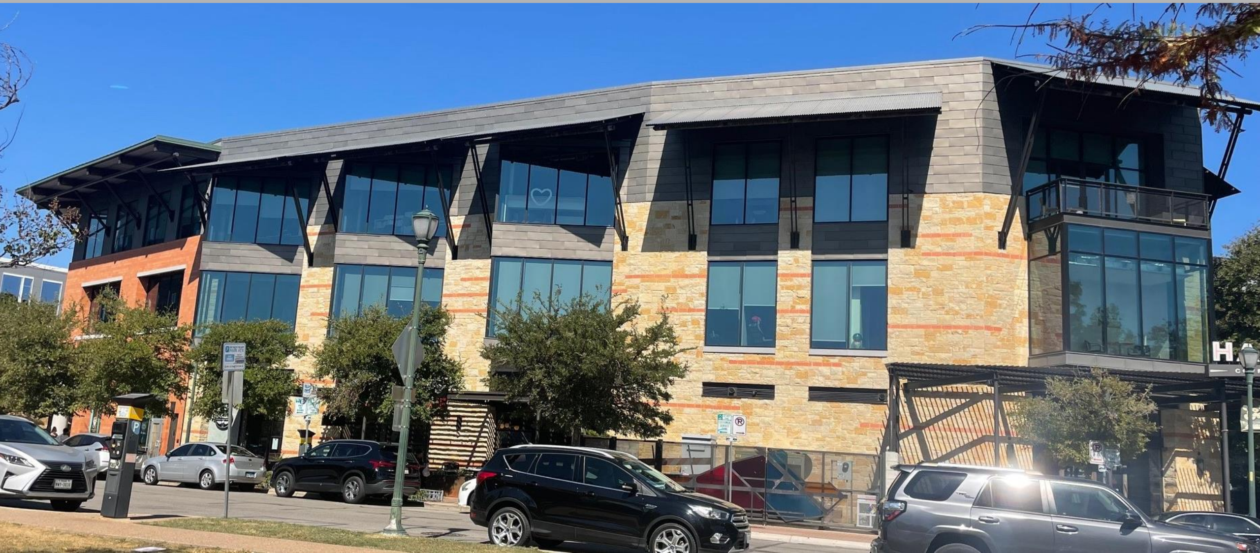
South, SW Elevations; 3pm September 29 th ; Austin, TX
