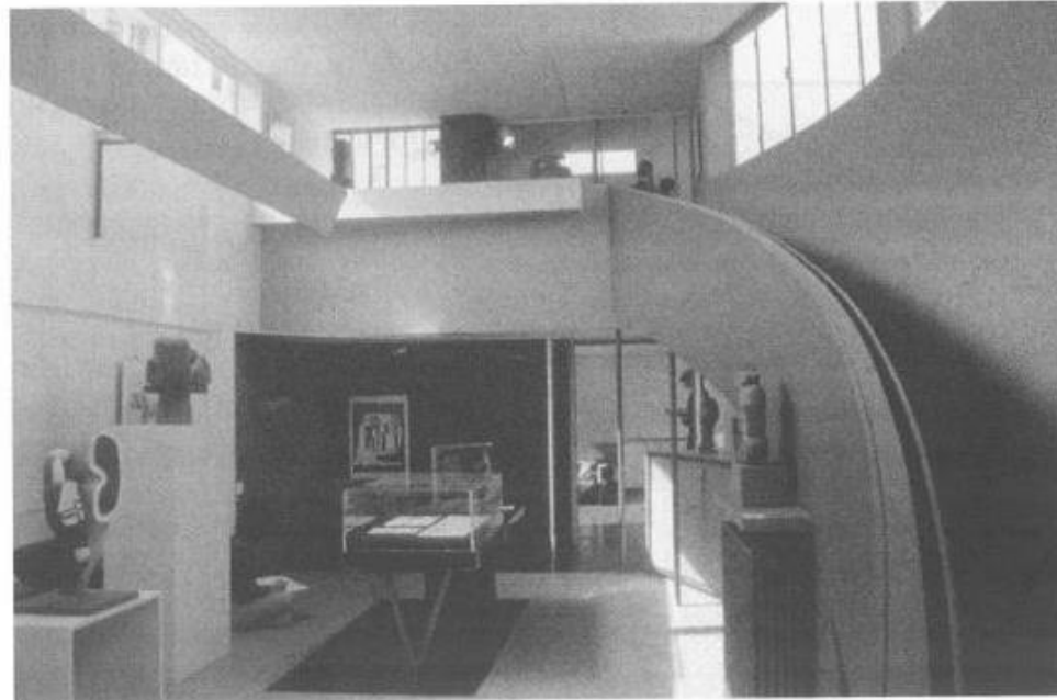
Figure 13.10c Strip or ribbon windows, as seen here in the Maison LaRoche by Le Corbusier, admit uniform light, which is further improved by placing the windows high on the wall. Note that photographic film exaggerates brightness ratios. (Photograph by William Gwin.)
