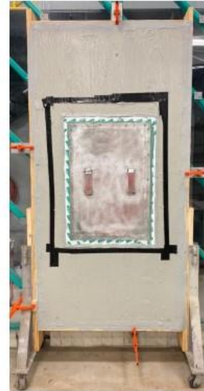
Wall 1 prior to the 4" ExoAir 110AT being applied
