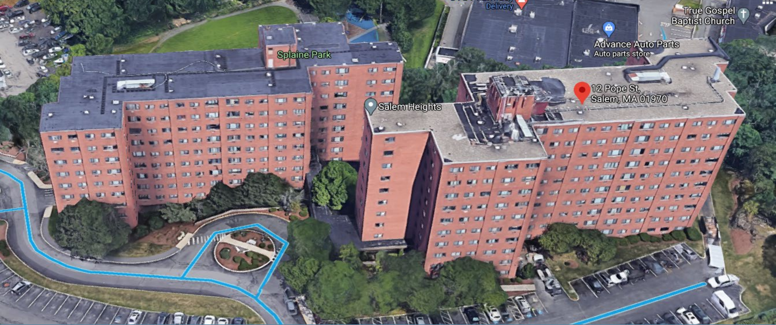
Salem Heights, 281 Units Family, Salem, MA Built: 1974
