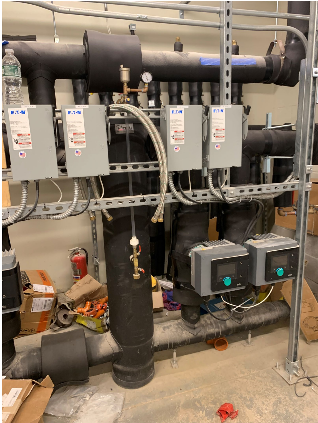
Geothermal Manifold
