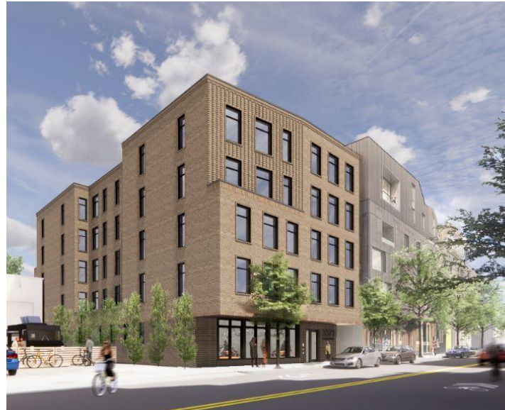
3371 Washington St. Boston, MA | 39 Units Phius Design Certified, In Construction
