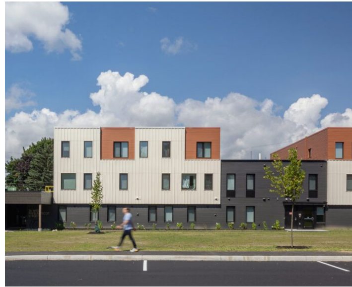
Front St. Portland, ME | 100 Units Phius Certified (Building 2), Design Certified (Building 5)
